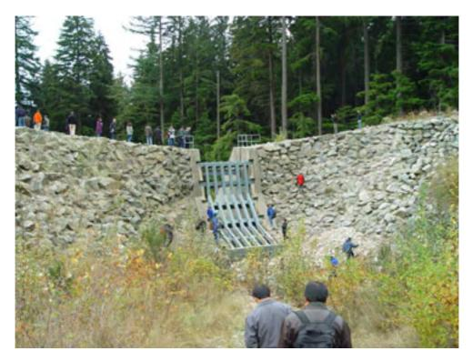
**Figure 6.0.1** A debris-retention outflow structure in a sediment-storage basin protecting a northern suburb of Vancouver, Canada. This structure is intended to safely stop events occurring about once in 500 years. To retain this capacity, the basin must be maintained relatively free of debris, and would be cleared after each significant sedimentation event even when these were not debris flows. There is a service road to access the basin for sediment removal.
