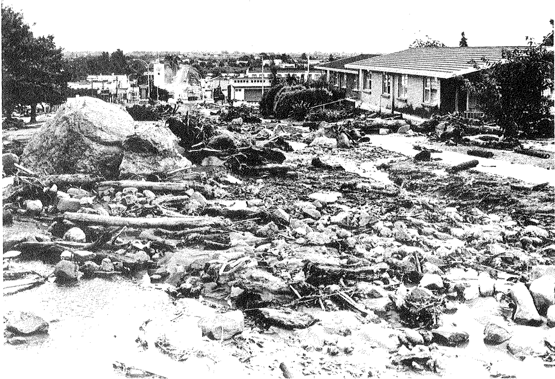
Fig. 2. Boulders and logs left in the path of the flood which swept away houses in Te Aroha. 'Auckland Star' photograph.
