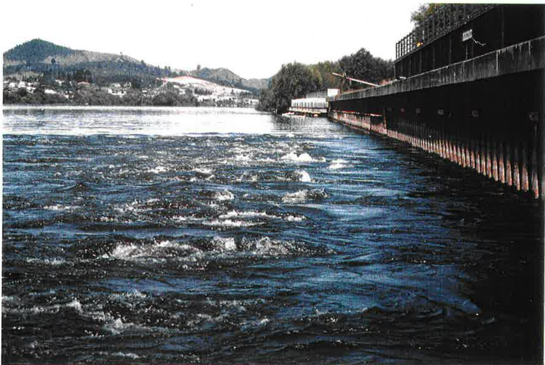
Plate 2. Upstream view of the Huntly power station outfall after the outfall ports were extended. Note low turbulence close to wall.
