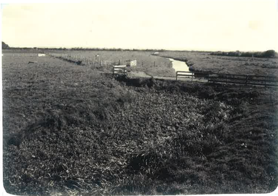
FIGURE 2. Drains showing weed removal by grass carp (above bridge) and their condition without grass carp (below bridge).
