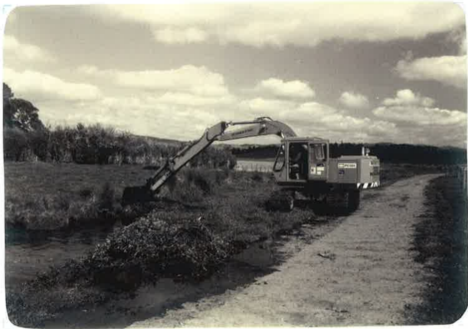
FIGURE 3. Draglining of a drain, showing the deposition of weed debris along the banks.
